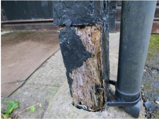
The columns of the porch of the village hall have deteriorated to the extent that at some point they will need substantial repair. They have clearly been repaired in the past but the wooden posts have been set into the concrete – they would be better fitting onto a raised stone base so that rainwater runs off them.
